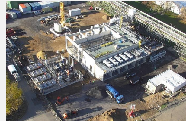
A 10 MW RefHyne electrolyser construction to be completed in mid-2021, Germany
